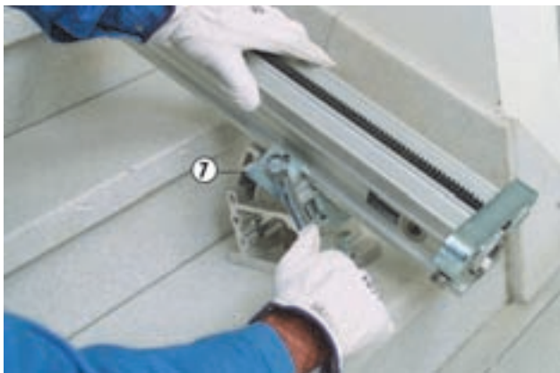
Installation of rail supports for angular cutting and cutting on stairs
