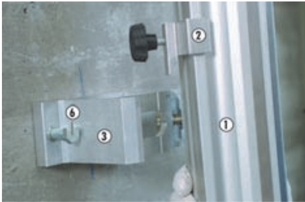
Installation of standard rail supports
