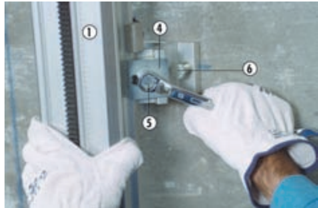
Installation of standard rail supports
